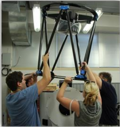
Installation of the Secondary Mirror Truss
